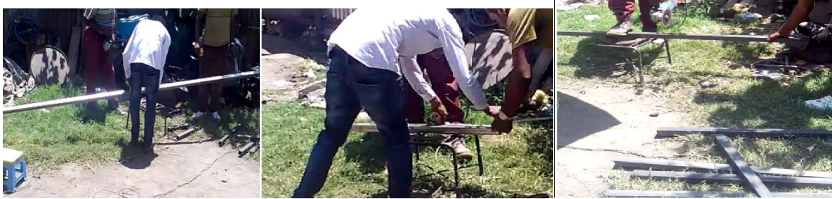
Figure 3.17 performing operation with appropriate material and equipment
