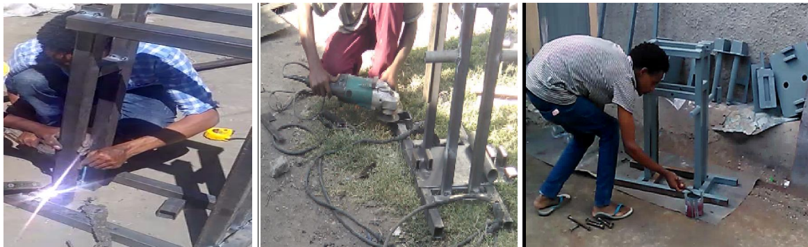
Figure 3.18 Joining, grinding and painting operation
