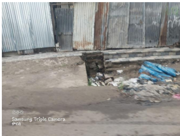
Fig 14. Blocked Drainages
