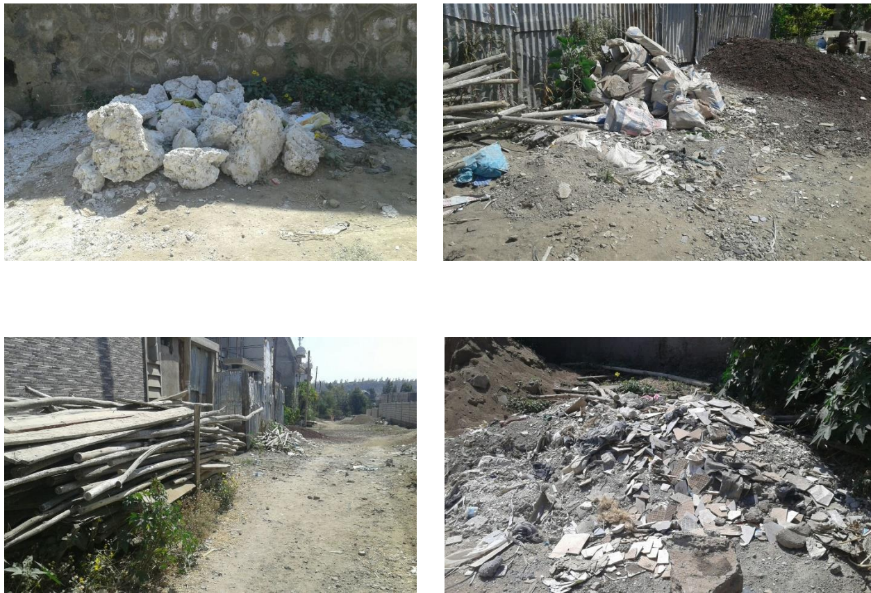
Fig 13. Construction waste disposal on streets
