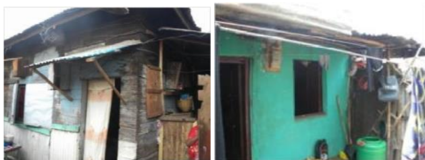
Figure 17 The residential area before the redevelopment
