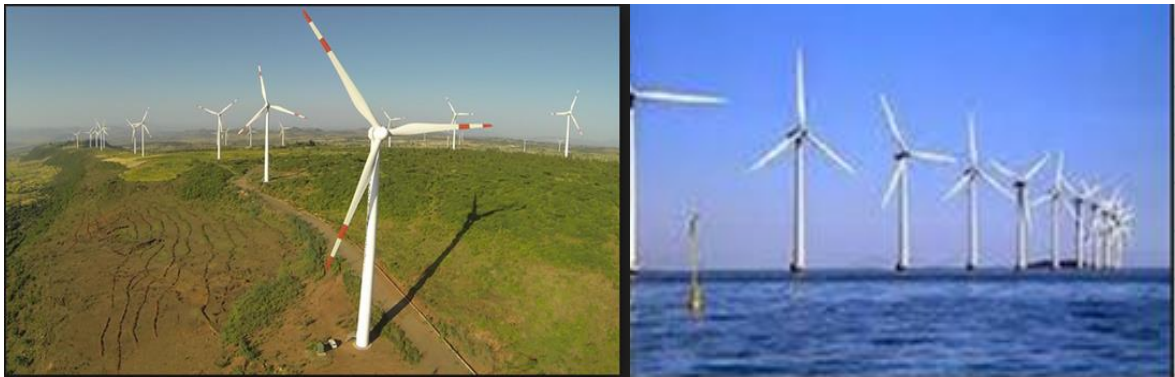
(a) Onshore Adama-I wind farm
