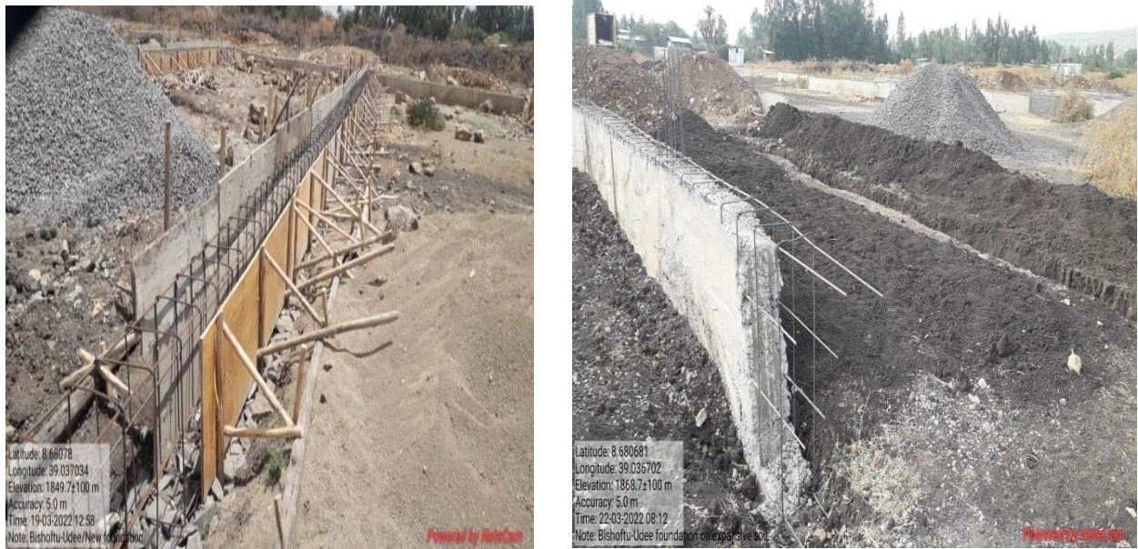
Figure 4. 16: Plinth beam foundation for G+0 buildings
