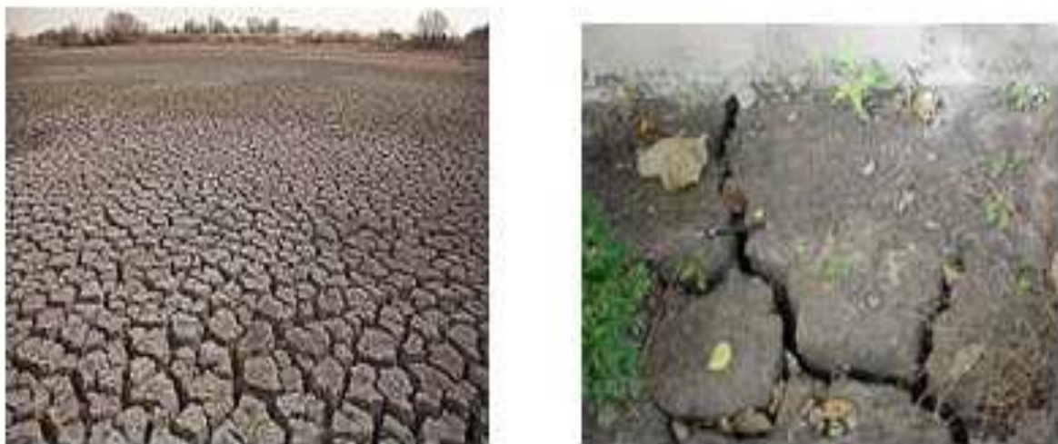
Figure 2. 2: Views of expansive soil with polygonal pattern of surface cracks in the dry season (Chen, 2018).
