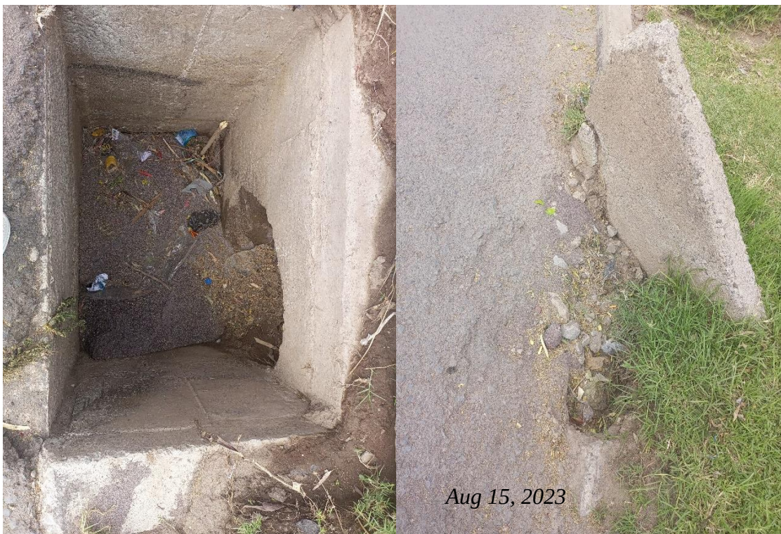
Appendix Figure 4. pictures of closed storm drains by dirt's, solid wastes and soil
