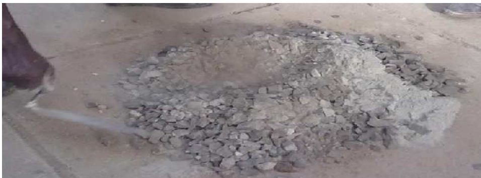
Fig.3.16. Dry mixing of the ingredients
