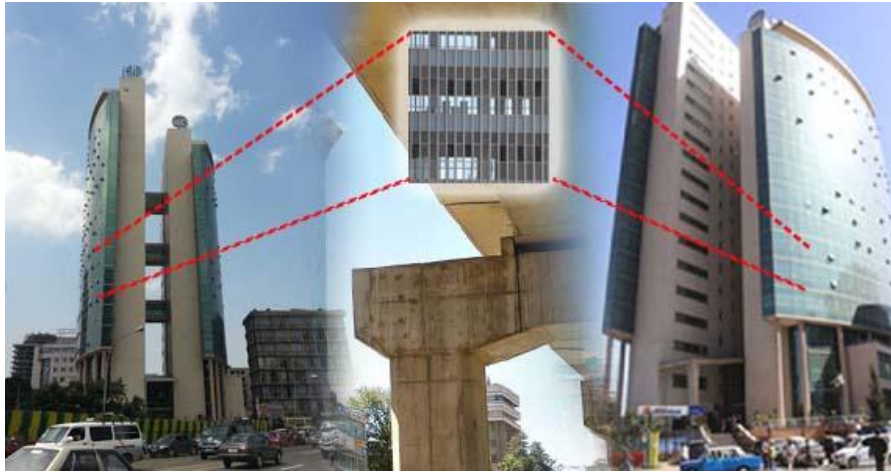
Figure 50 Awash bank building envelope (Source: Site Observation Author 2024)
