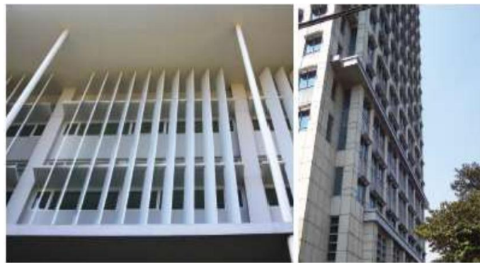
Figure 15 Example of the Vertical Fins Application (Mansouri, 2023)
