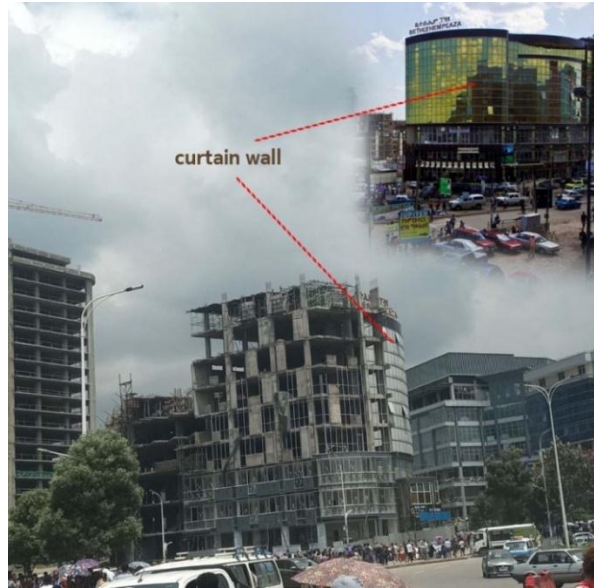
Figure 46 Bethlehem plaza building envelope (Source: Site Observation Author 2024)
