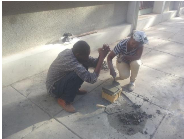
Figure 3.6 placing concrete mix
