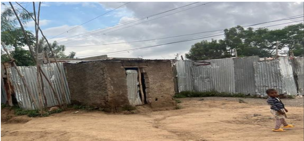
Figure 4. 3: Low-Income Group of Peoples Un-able to Re-build their Houses
