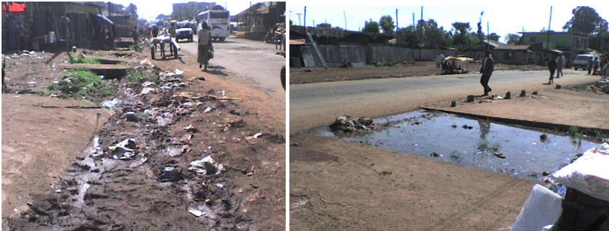
Figure 4.22 Ditches filled with silt and solid wastes and rain water collected in parking's and walkways (Source: photo by the author, 2023)
