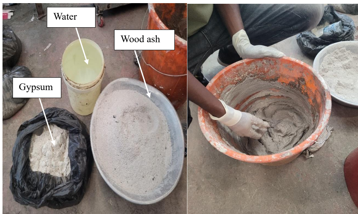
Figure 4.7 Preparation of the insulation material.
