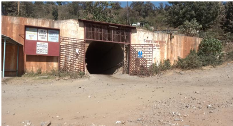
Fig1.1 East Sakaro Underground Tunnel ( Derartu jibro, March 2022)
