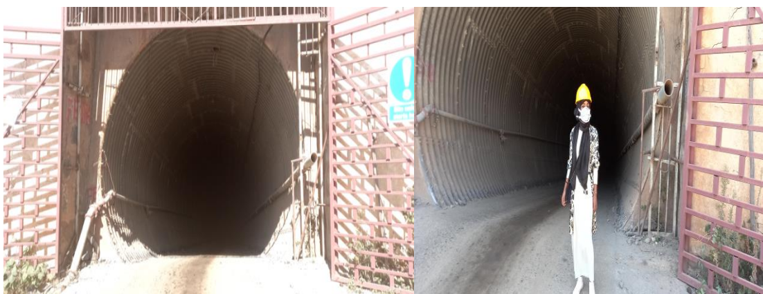
Fig5.1 Portal gate of a tunnel for Sakaro underground gold mine (Derartu jibro, March 2022)
