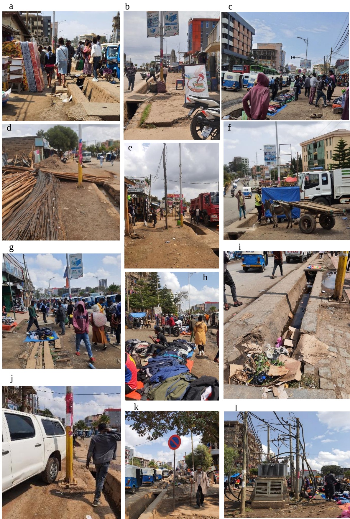
Figure 5:Overall status of street. Blocked sidewalks (a,b,d j,f),utility lines (e),vending (h,c) Congested sidewalk (g), damaged ditches (i), transformer on side walk (l), elderly person (k)
