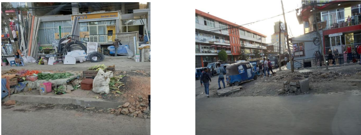
Figure 9 Unsafe for people with disabilities
