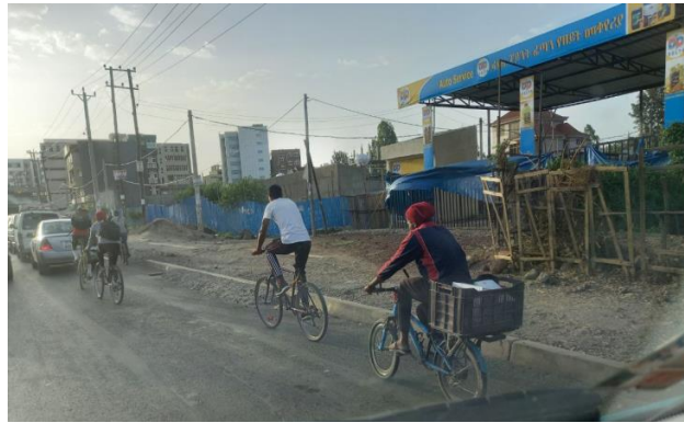
Figure 12 Lack of cycle lane
