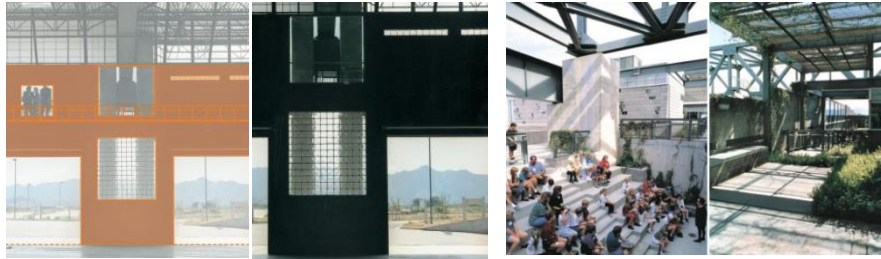
Figure 7: Elevated Public Pedestrian Pathway and Industrial Transparency: Large Windows, Sky Lights, and Glass Blocks
