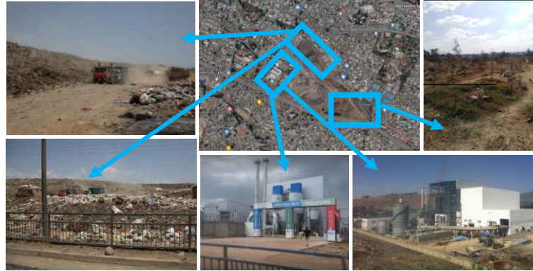
Figure 3: Waste to Energy Plant, Dump Site, and Closed Part of Reppi
