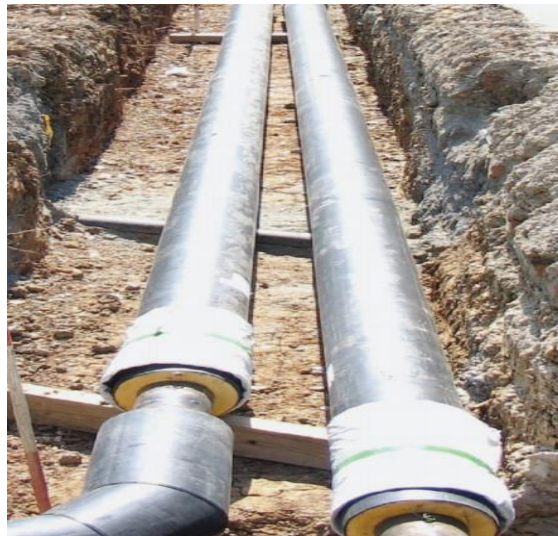
Figure 37: Buried pipes installation (Sanja et al., 2011)
