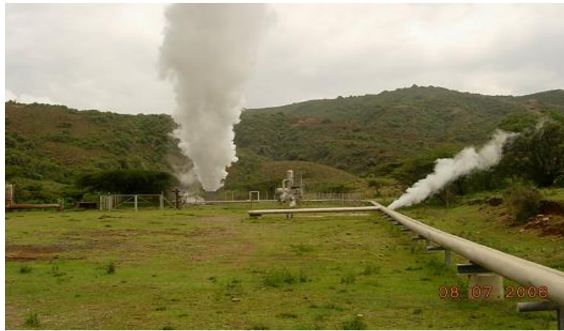
Figure 14: One of the discharging wells (LA-3) of the Aluto-Langano Geothermal Field, total depth and maximum temperature of 2.3 km and 320°C, respectively (Kebede et al.,2010).
