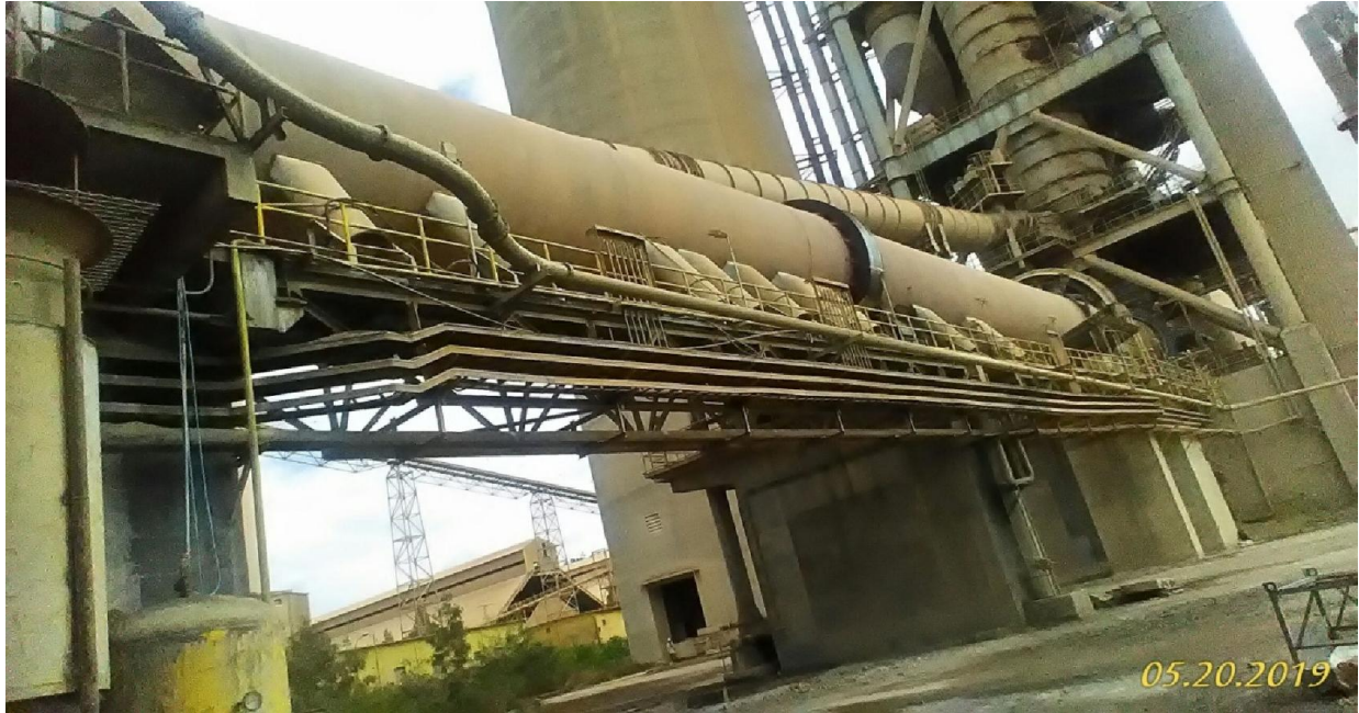
Figure 3.2 Photograph of rotary kiln
