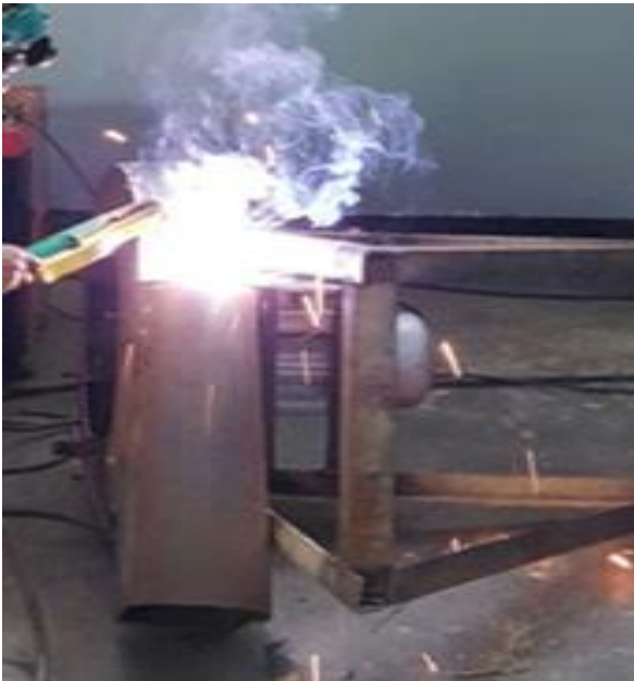
Figure 3. Welding of housing
