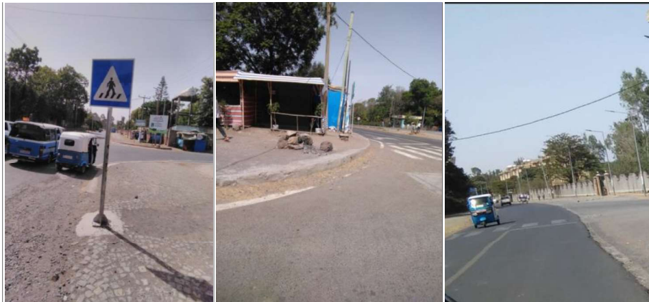
Figure 4.14: Pictures illustrate the street crossings conditions;
