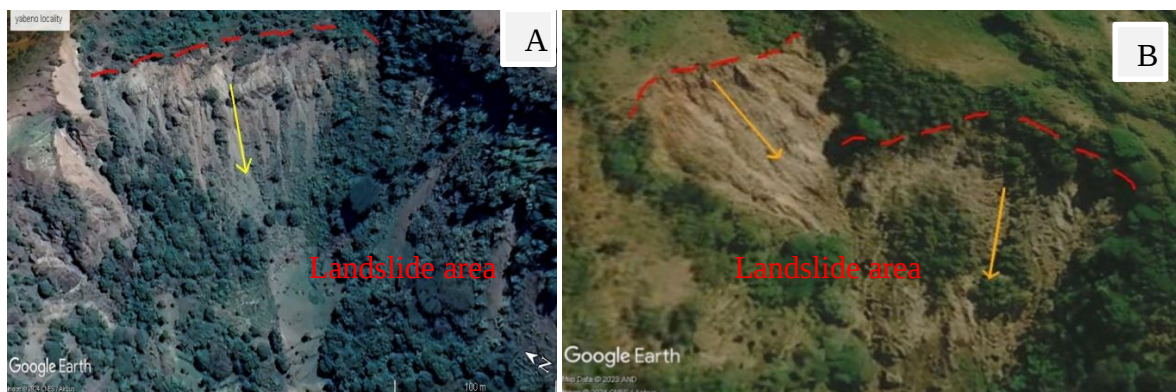
Plate 2. A) Rock unit sliding down, B) creep types of landslide (Google Earth Pro) in the Yabeno locality is made up of strongly and weathered basalt and is located close to the foot of a steep slope.
