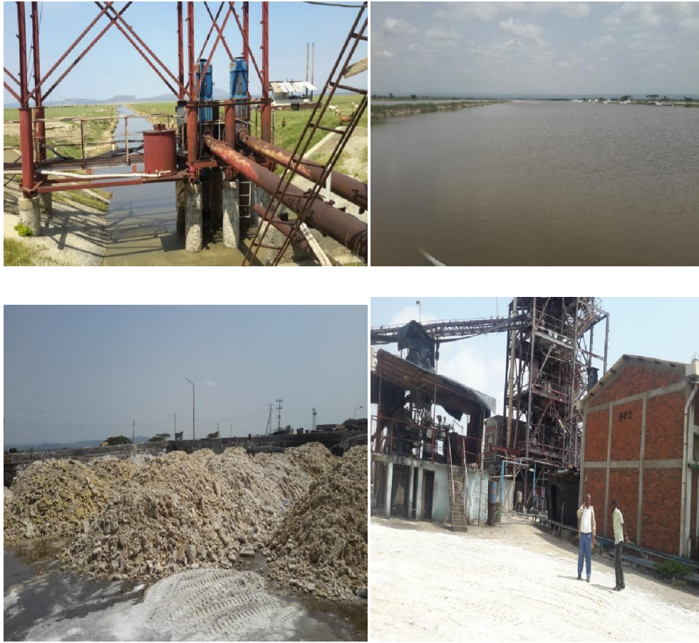
Figure 4.4: Partial View of Abijata-Shalla Soda Ash Plant
