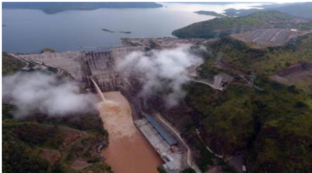
Figure3.2-Gbee III hydropower plant dam
