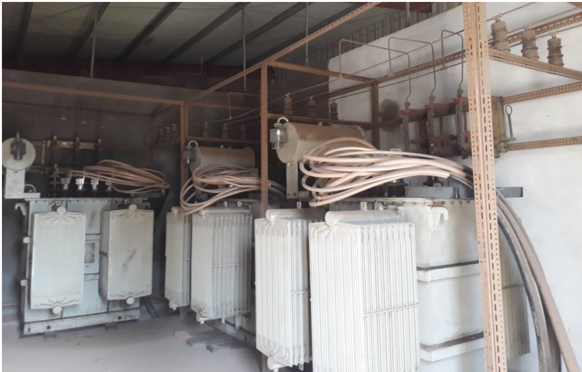
Figure.1. 2.Powerhouse of the Adama Spinning Factory seen in part
