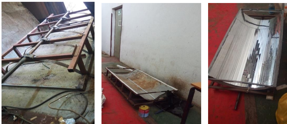
Figure 4.14: Construction of PTC and Reflective Mirror
