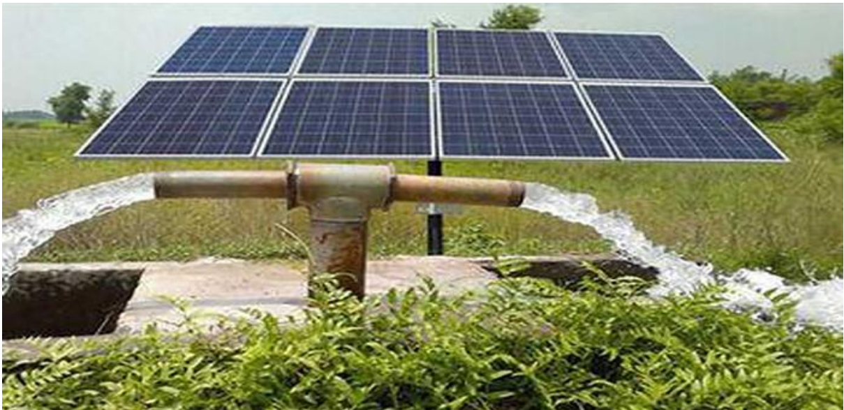
Figure 2.1: Village water supply West Madison (Source:acellcsolar Solarirrigation)
