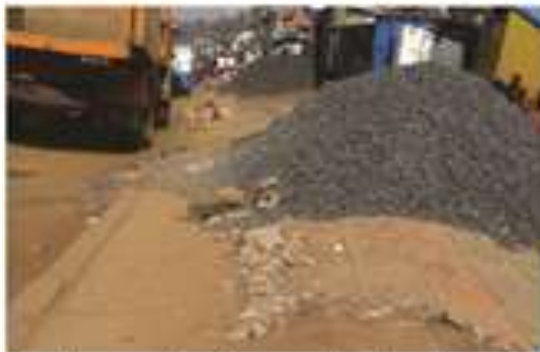
FigA: construction materials dump
