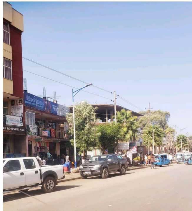
Figure 17 commercial buildings type
