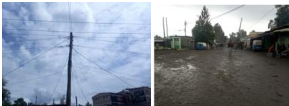
Figure 12 Lighting system on the site
