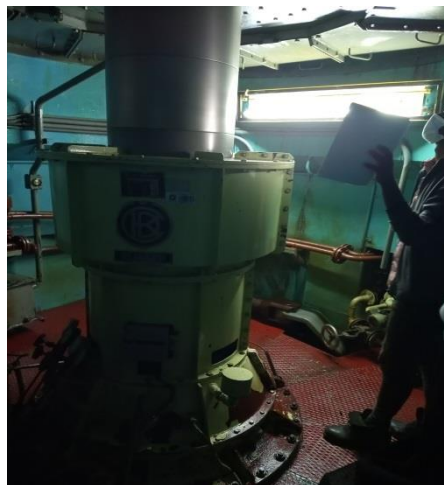
Figure 1.3 Francis Turbine covered with its housing.
