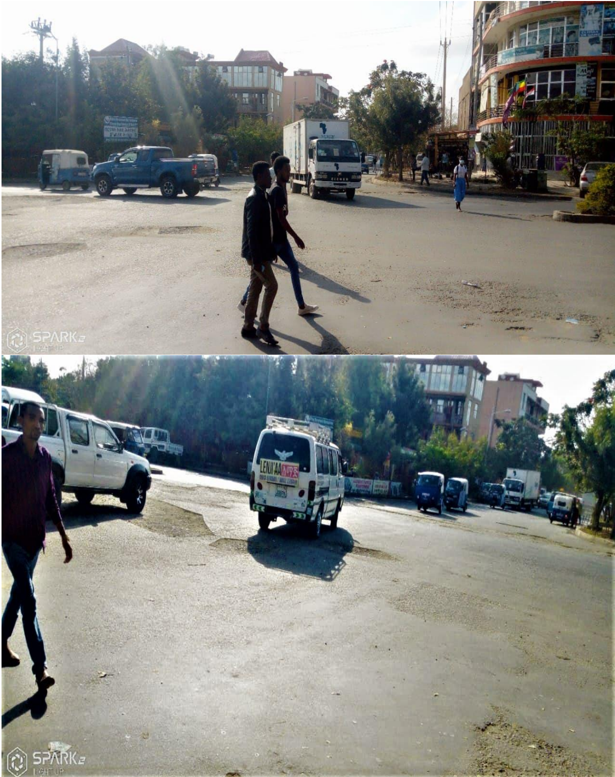
Figure C.6. Photo no zebra crossing, no pedestrian crossing, no properly constructed side walkway at 04 Condominium.
