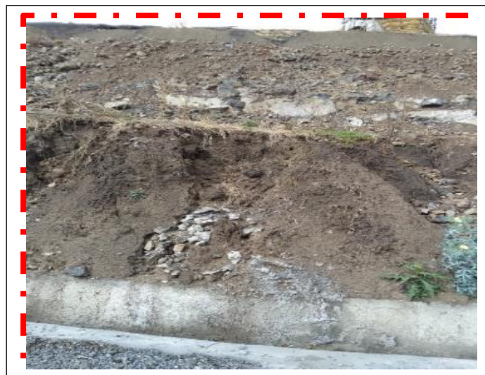
Figure 3. 4: Residual soil affects by erosion with at top basaltic rock
