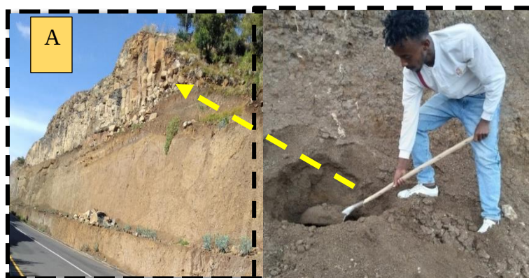
Figure 3. 4: Residual soil affects by erosion with at top basaltic rock
