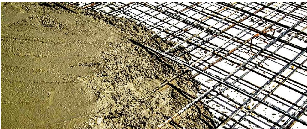
Figure 8: Steel reinforcement mesh concrete work of Bio-digester with 20cm wall thickness
