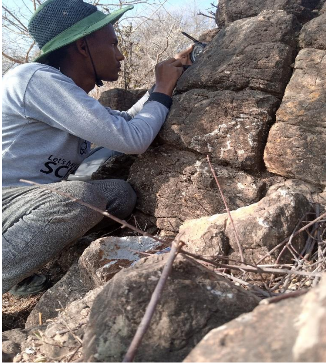
Figure 4. 3 Rhyolite exposure from downstream of left abutment
