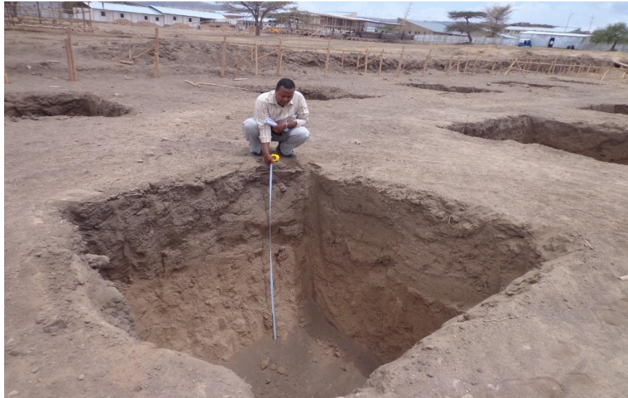
Fig. C.1 The profile view of Pit for the specimen TP 3
