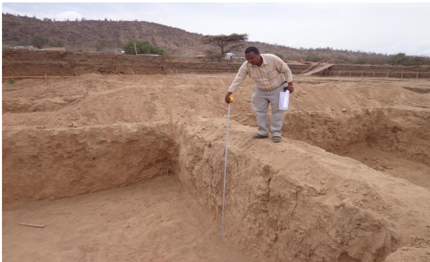
Fig. C.4 The profile view of Pit for the specimen TP 10
