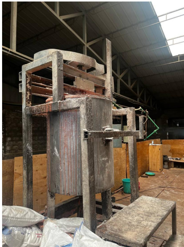
Figure 17: Adhesive mixing at the plant (Source: Author, 2025)
