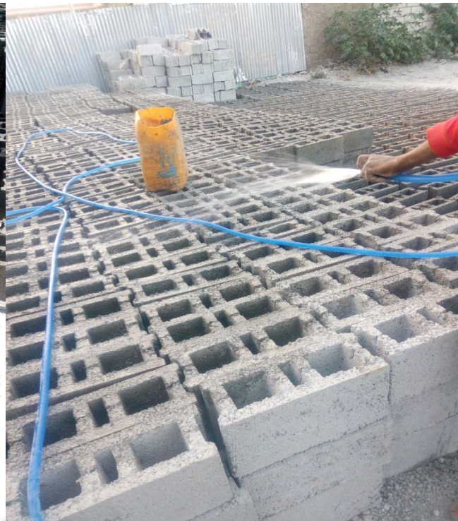
Fig. 5.11. curing process by sprinkling tap water around Cherkacherk
