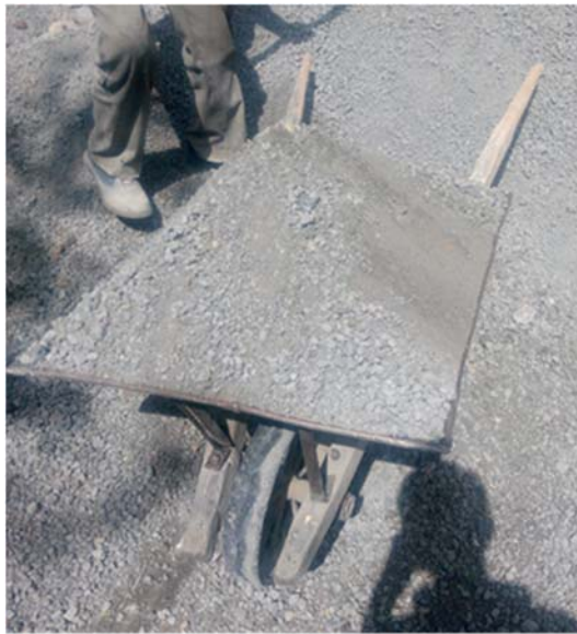
Fig. proportioning using wheelbarrow at gendegara site (res. 01)
