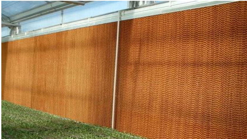
Figure 2.8 Fan and pad greenhouse evaporative cooling system [21]
