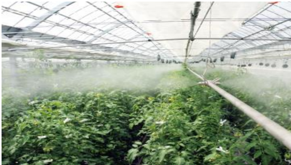
Figure 2.9 Fogging system for cooling a greenhouse [24]
