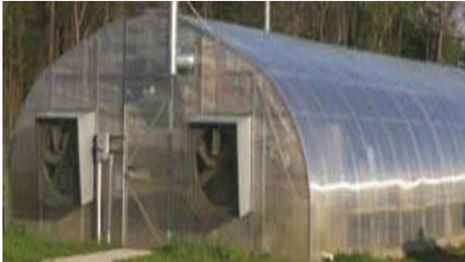
Figure 2.2 Quonset Type Greenhouse [10]
