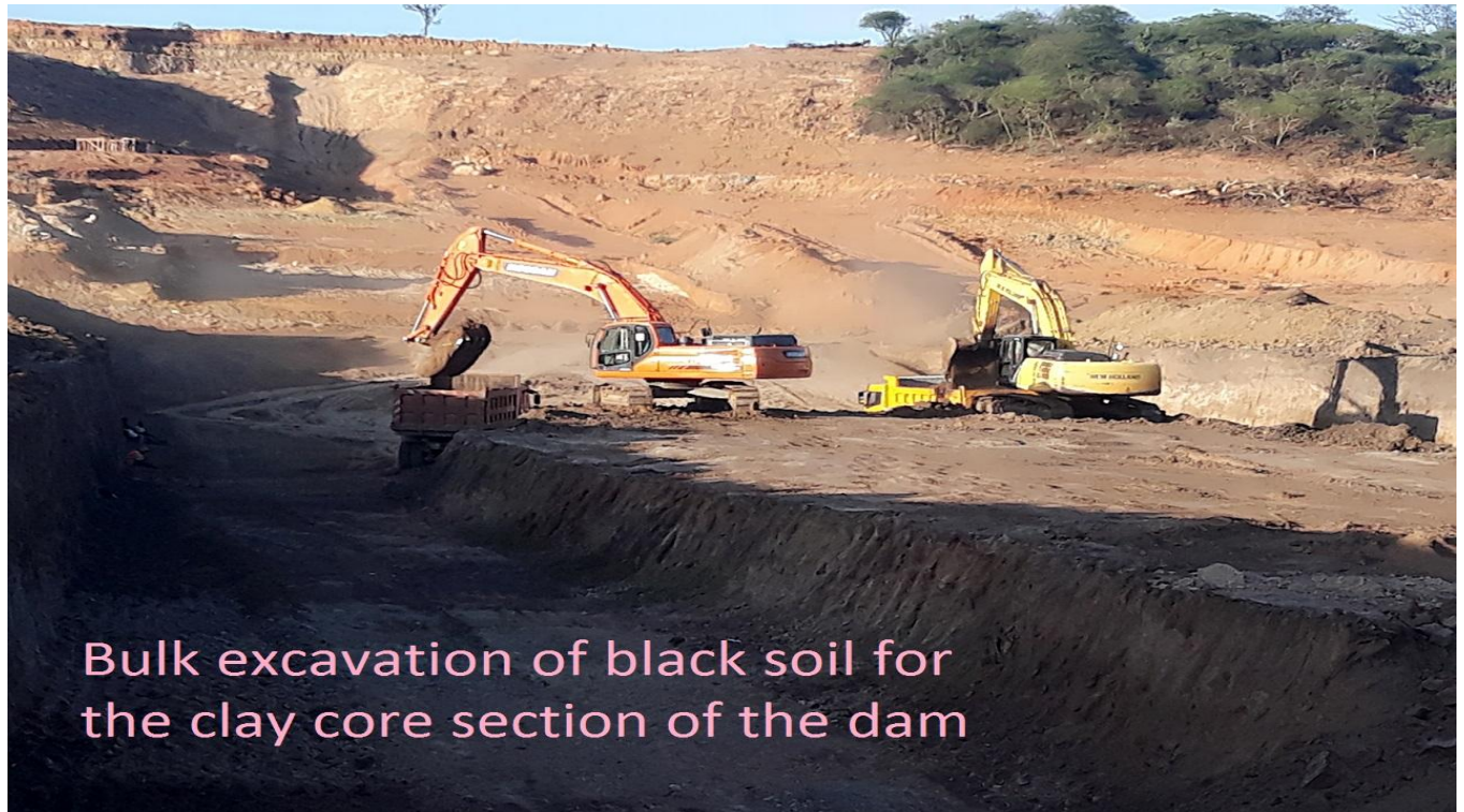
Figure 3.9: Clay core section excavation and preparation
