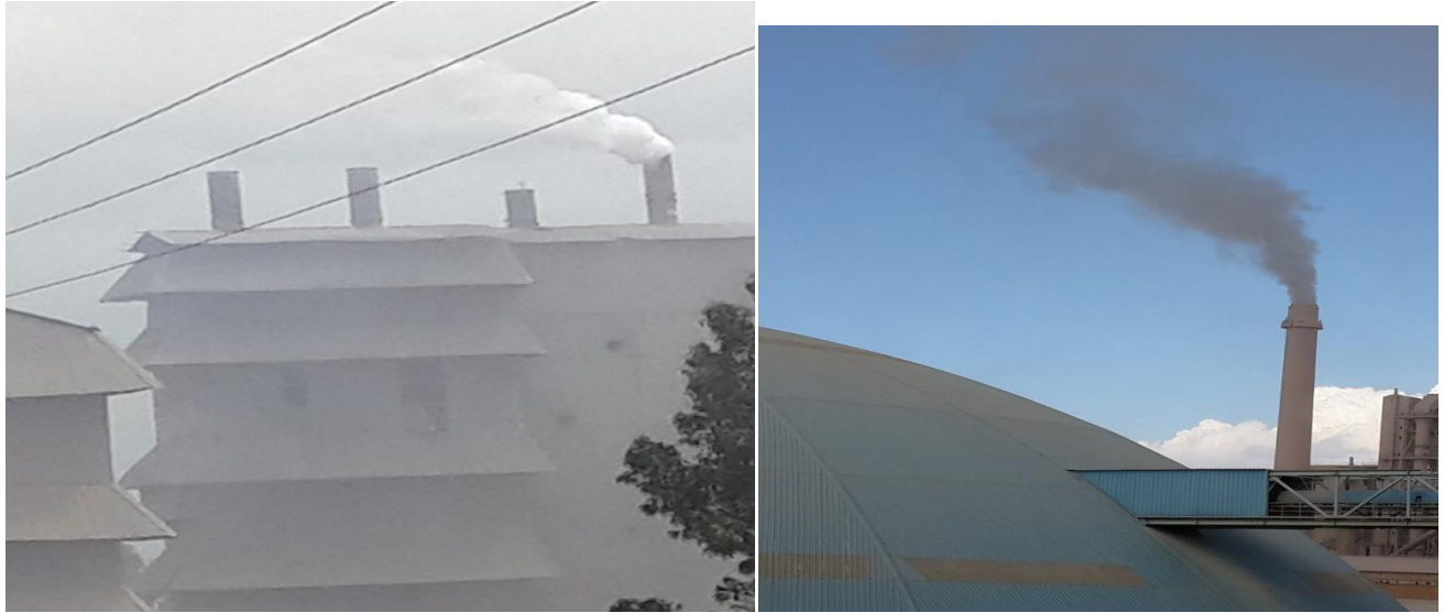
Annex picture1: Dust pollution from Abyssinia and Mugher cement factories
