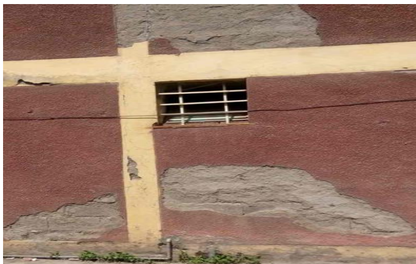
Figure 4. 7: Timely repairs and maintenance
