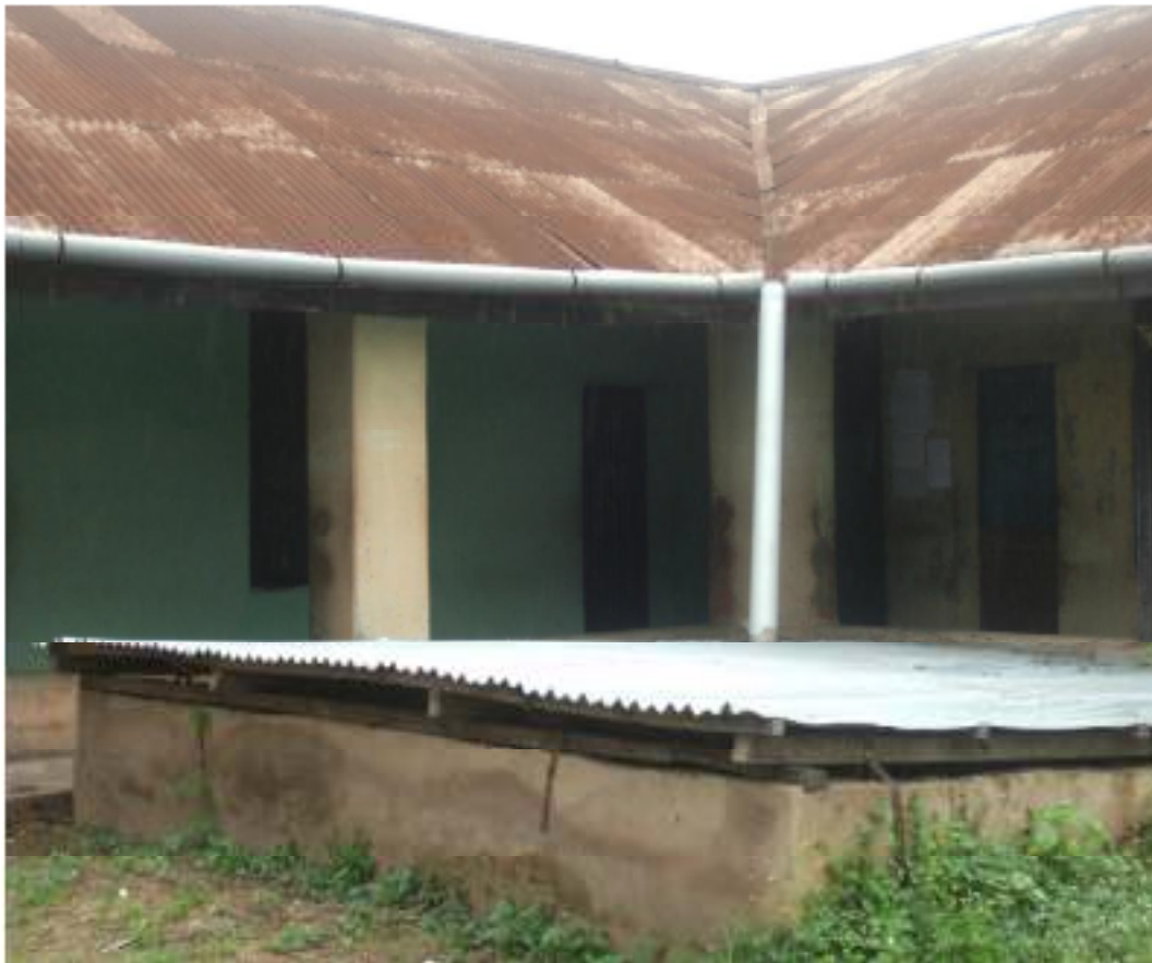
Figure 2.3: Roof catchment system (Oyewumi, 2013).
