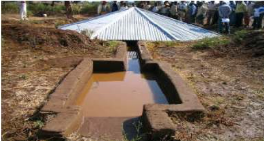
Figure 2.6 CIS roofed pond (Yusuf and Kiyoshi, 2006).
