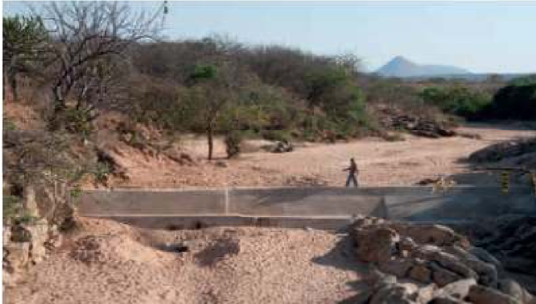
Figure 2.5: Sand dam (Mekdaschi and Liniger, 2013).
