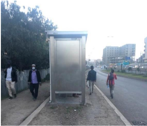
Figure 4.2.3: Bus station shade
