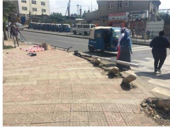
Figure 4.2.2 Pedestrian way at street junction
