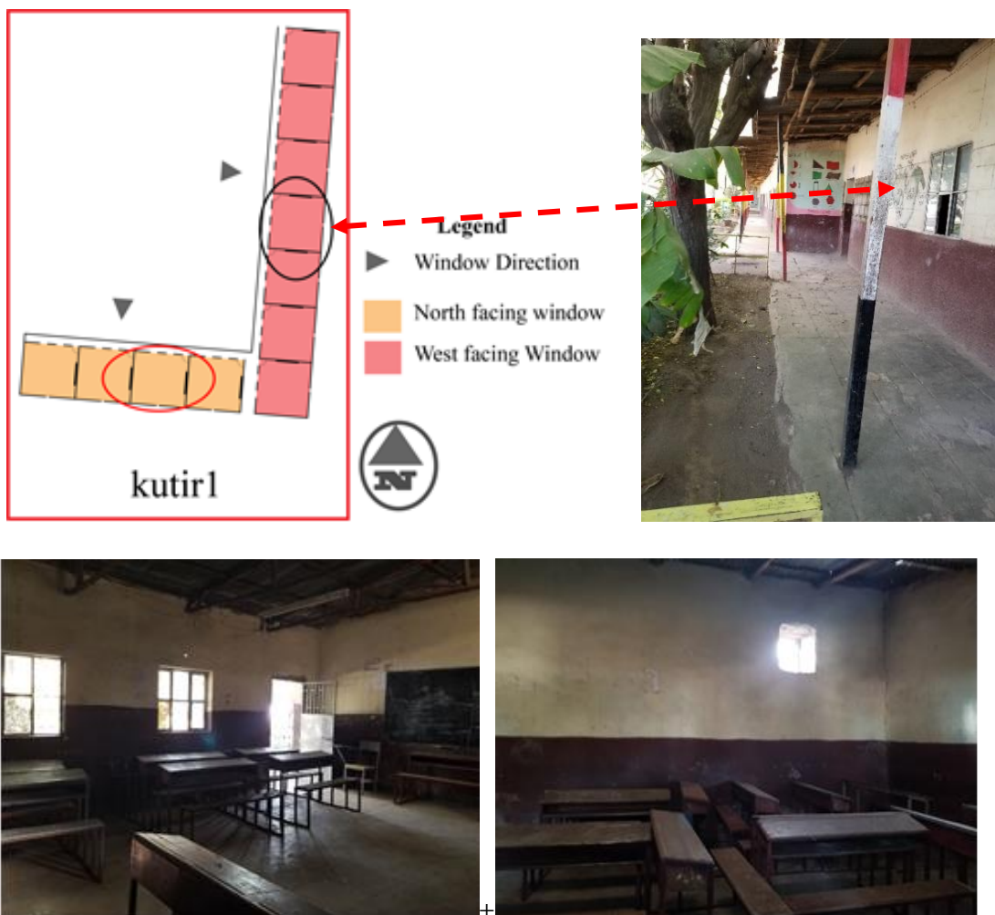
Figure 7 Kutir 1 classrooms orientation and field image
