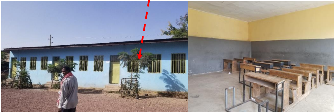
Figure 25 Kidus Quran classrooms orientation and field image
