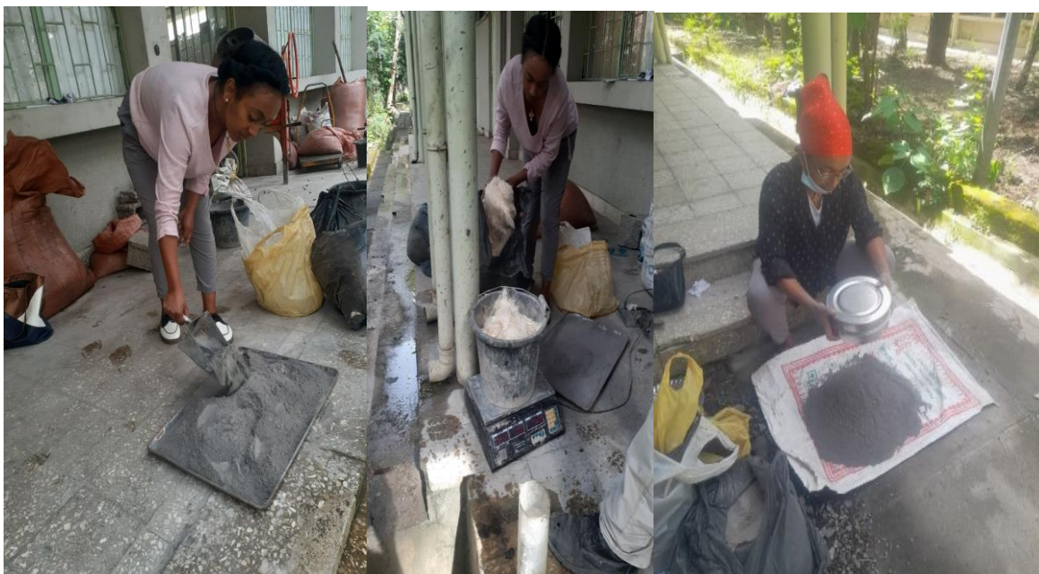
Figure H 6 Measuring and preparation of material for mixing
