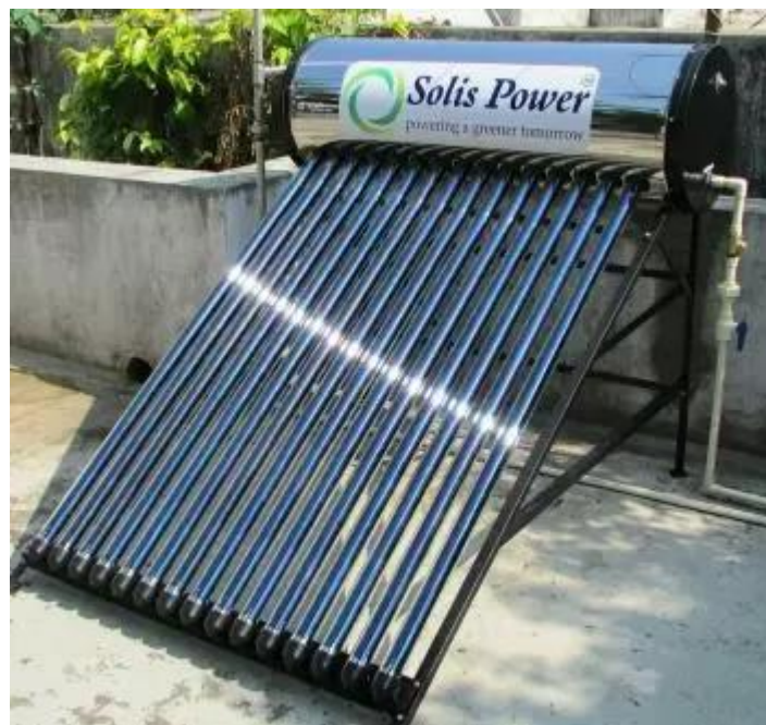
Figure 2. 2 Thermosyphon SWH system (Dimitrios, 2001; Panapakidis, 2009)
