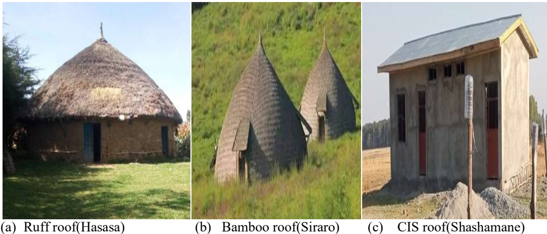
Figure 6: Roof cover type commonly used in West Arsi
