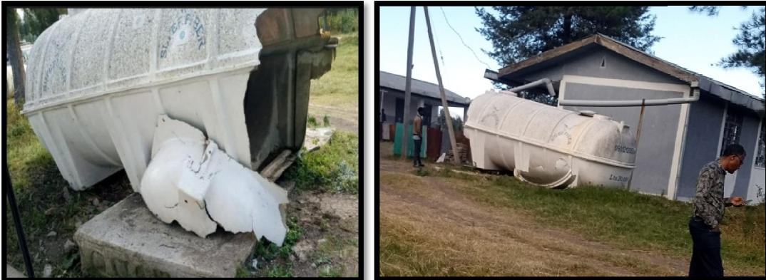
Figure 14: Destroyed storage tank and Connection at Observation point 4; September 2022
