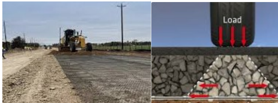
Figure 2.4: Geogrid inclusion while subgrade preparation (Archibong GA et al, 2020)
