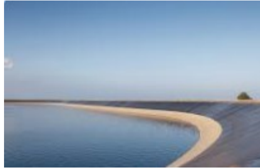
Figure 2.5: Geomembrane (Chatrabhuj et al, 2024)
