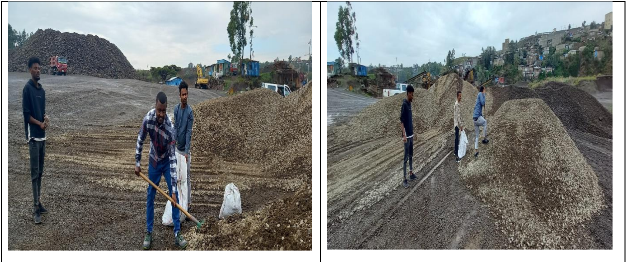
Figure 3.12 Sampling of Crushed Aggregate Base Course from Bulbula Crusher Site
