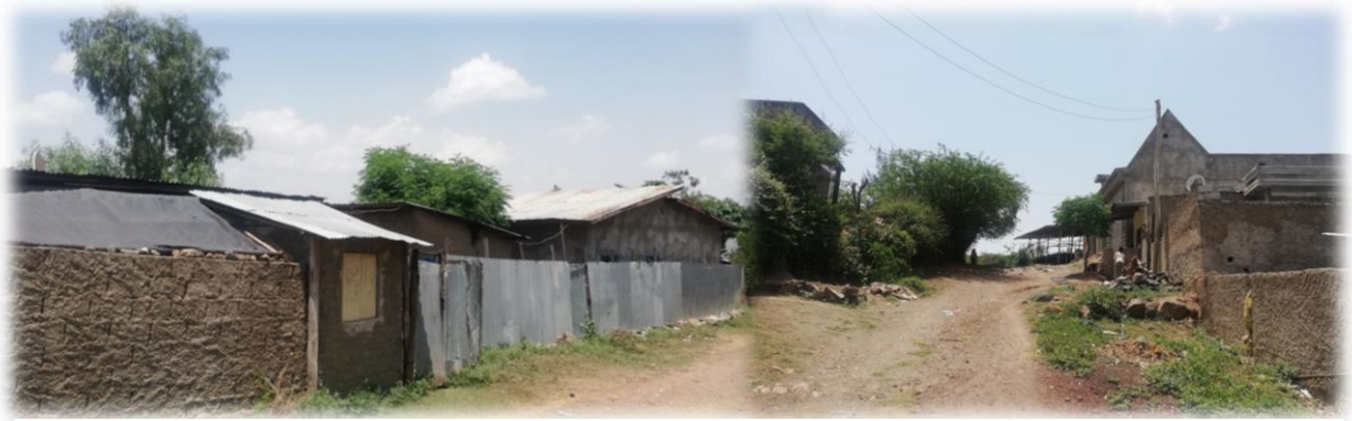
Figure 25 housing settlements in fair condition
