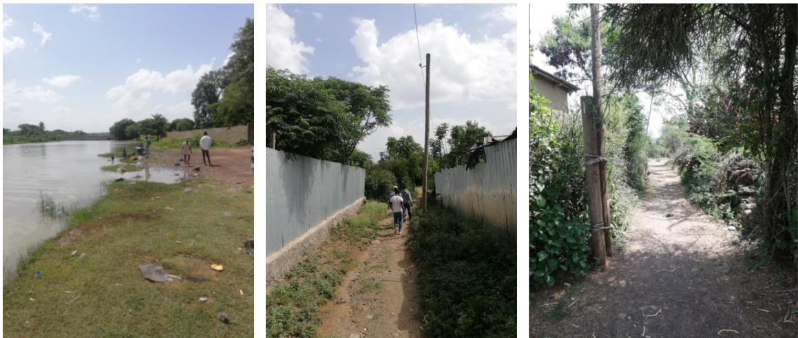
Figure 12 infrastructure condition of the town
