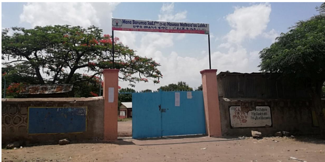
Figure 16 existing elementary school
