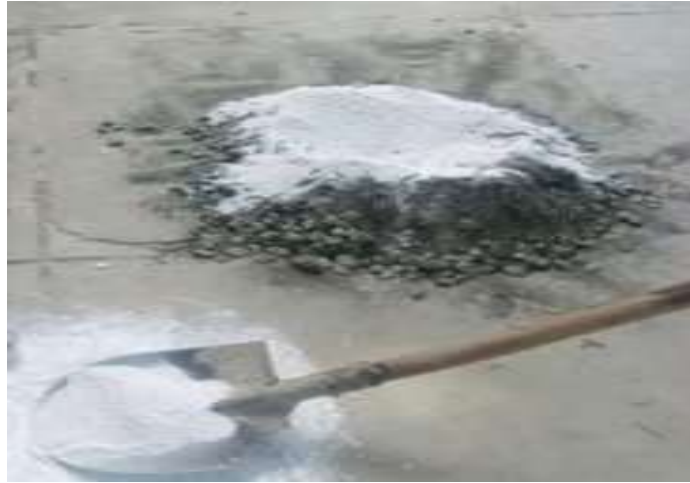
Figure 3.21 Hand mixing
